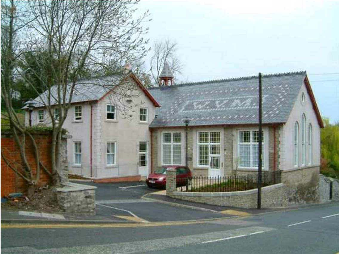
A good example of a restored BLI - St. Winefride's School, Holywell now converted to flats and called Plas Gwenfrewi (carried out using Townscape Heritage Initiative grant money)
